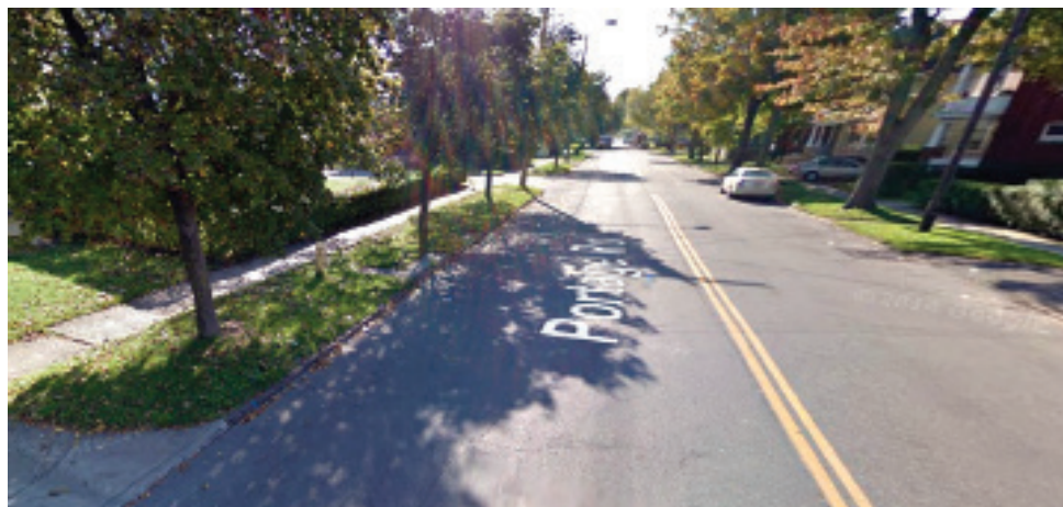
What lies under Portage Road? A test would find out conclusively.
